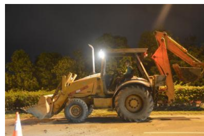
Gambar 51 : Jentera backhoe excavator .
